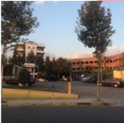
Picture 2 – Photo of site 2/6
