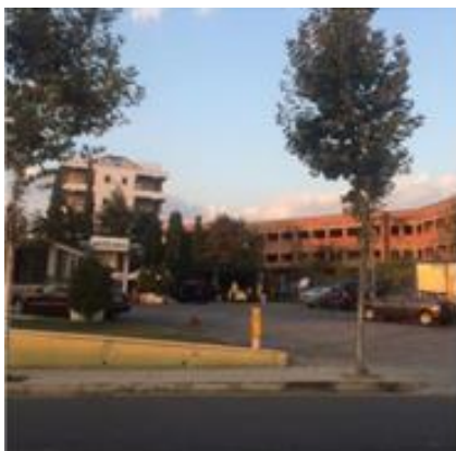
Picture 2 – Photo of site 2/6
